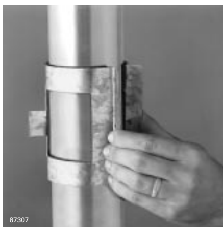
Figure 14 Install vent clamps on vent piping
