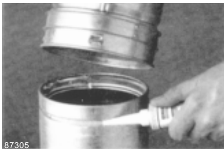
Figure 12 Sealing B-vent joints
